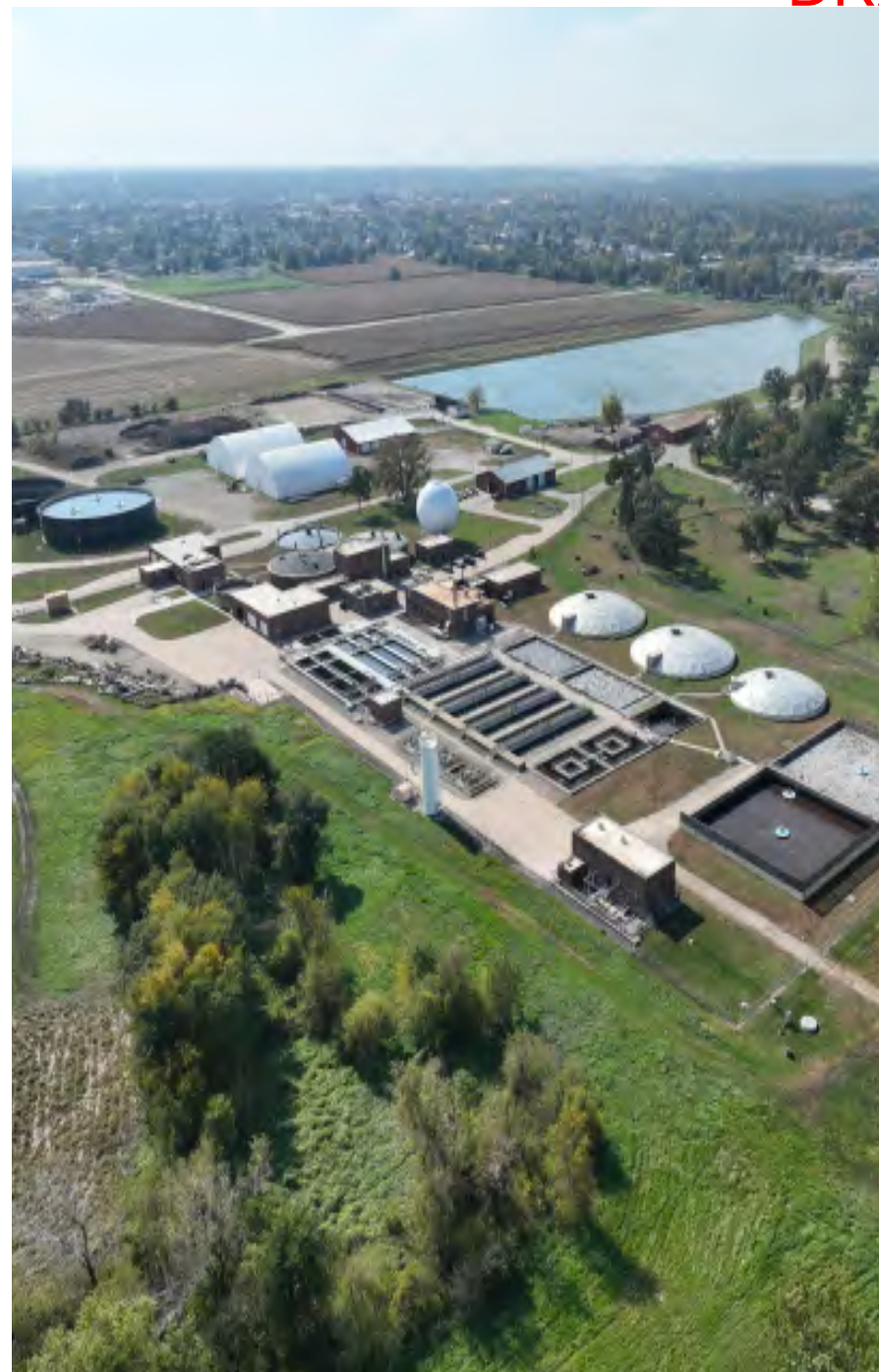
Marshalltown Water Treatment Facility
