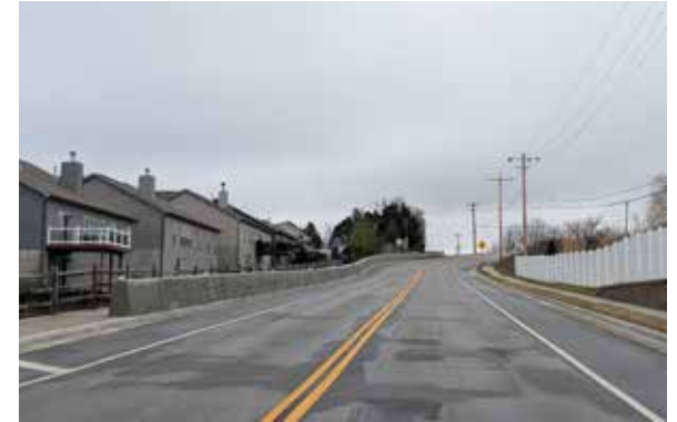
| Recently constructed sidepath and sidewalk along Duello Road
