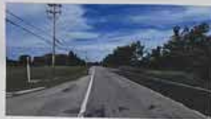
Roadway without trails or sidewalks.
