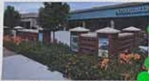
Brick border wall with integrated art panels
