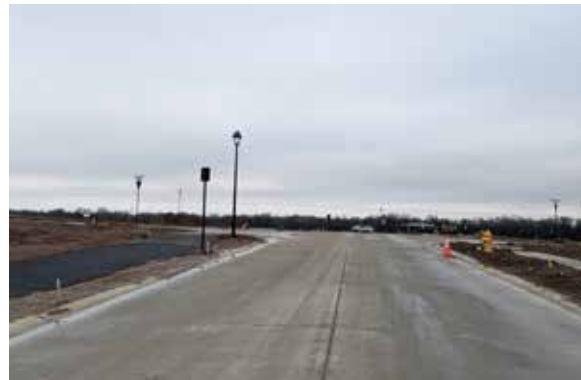
| A new sidepath and sidewalk have been constructed on Integrity Drive in the new Post Farms development
