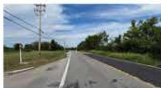
Roadway without trails or sidewalks.
