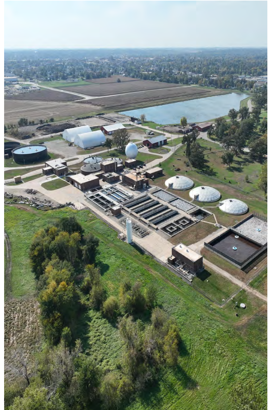
Marshalltown Water Treatment Facility
